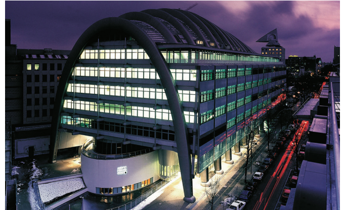
The Ludwig Erhard Haus building in Berlin, Germany
