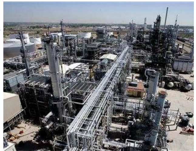
Manjoon Oil Field: The first project in Iraq for 30 years which adds substantial new oil processing facilities.
